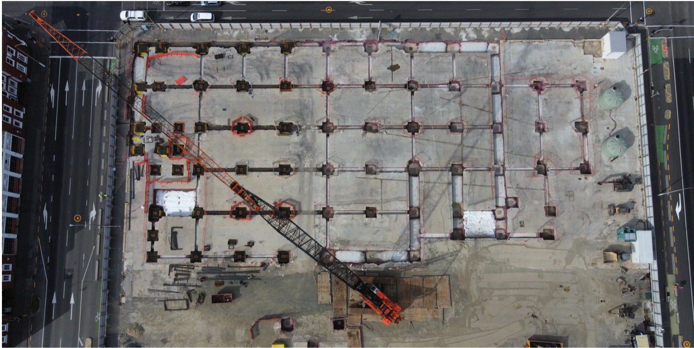
Birdseye view of the build site. Image courtesy of RCP
