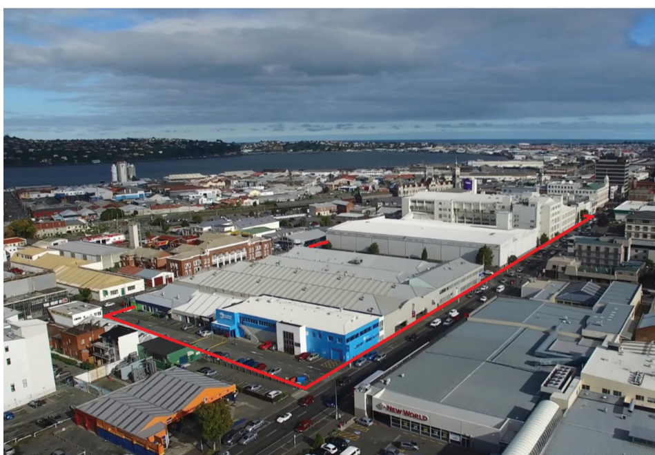
Looking Southbound at the Wilson's and Cadbury demolition sites
