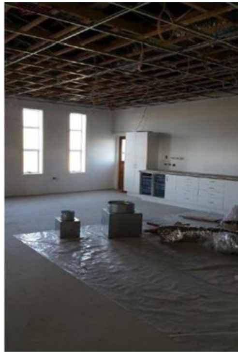
Above: Skills Lab showing new Joinery and Ceiling Grid
